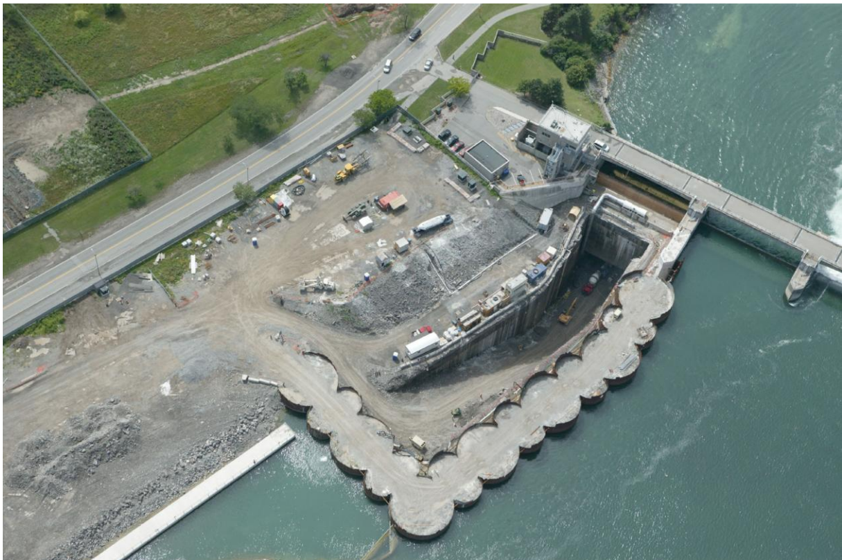
5 6 Photo 6 - Aerial of Intake Site Surrounded by Cofferdam
