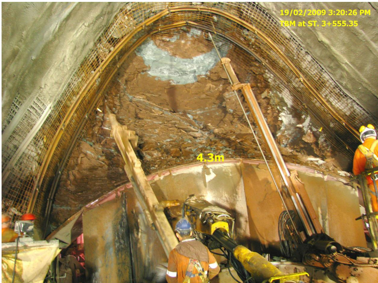
Photo 13 – Overbreak of more than 4 metres
