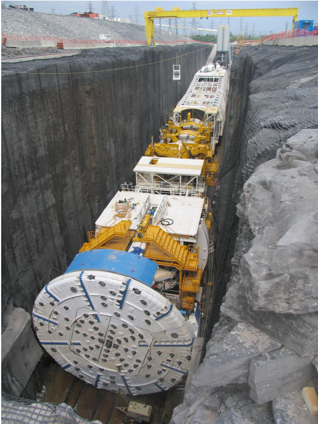
1 Photo 8 – “Big Becky” Assembled in the Tunnel Outlet Site Prior to Tunneling
