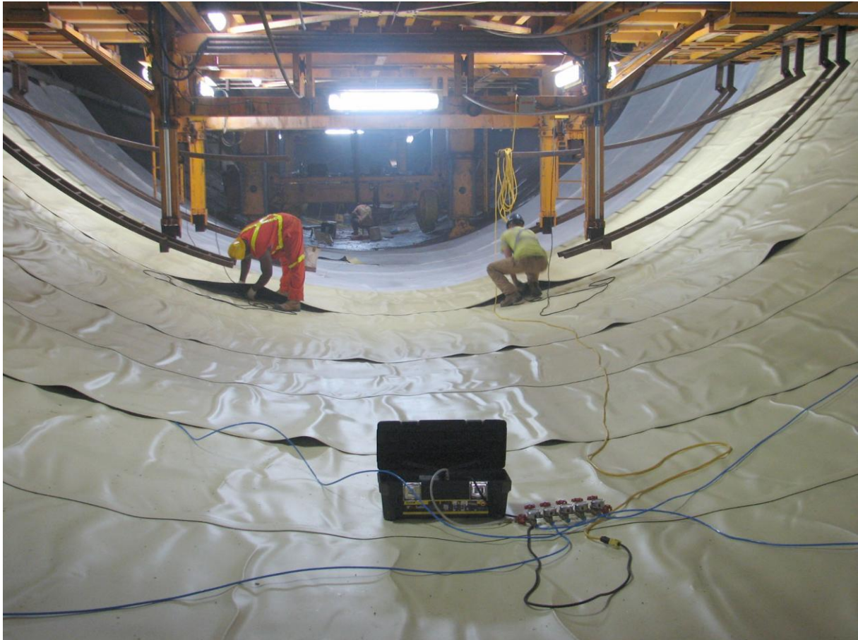
Photo 12 - Testing of the Invert Lining
