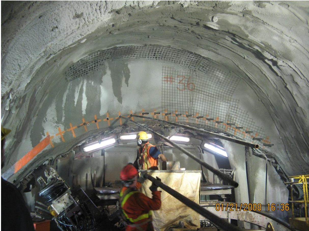
Photo 9 - Installation of Spiles in an Umbrella Formation
