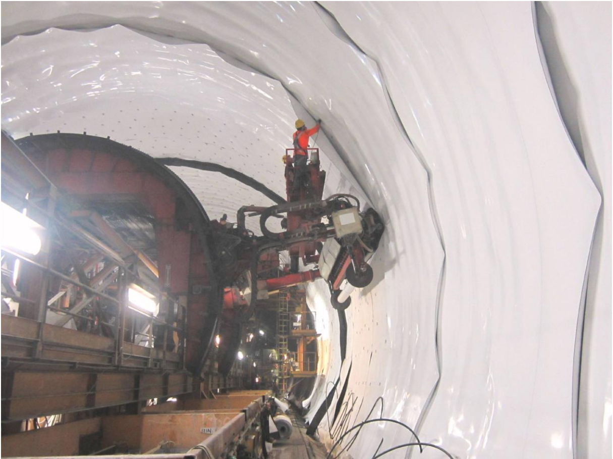
Photo 15 - Installation of Arch Membrane
